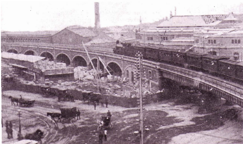
Above—Duplicating the viaduct to provide four tracks. Below—Constructing the first viaduct, opened in 1891.
