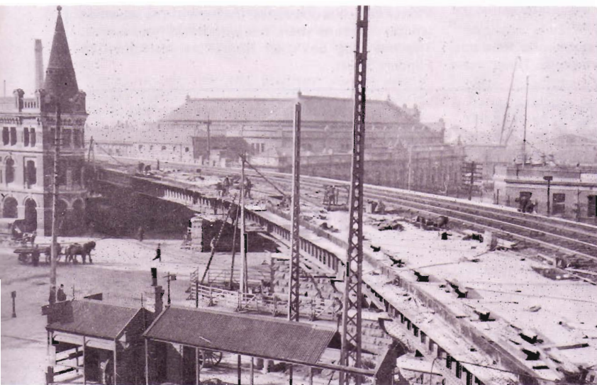
Above—Duplicating the viaduct to provide four tracks. Below—Constructing the first viaduct, opened in 1891.
