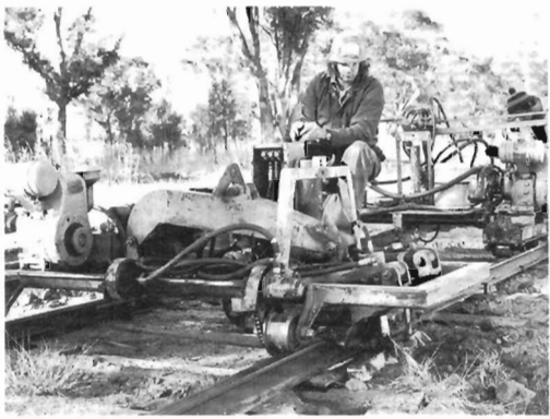
The first machine along the track is the rail-sprayer.
