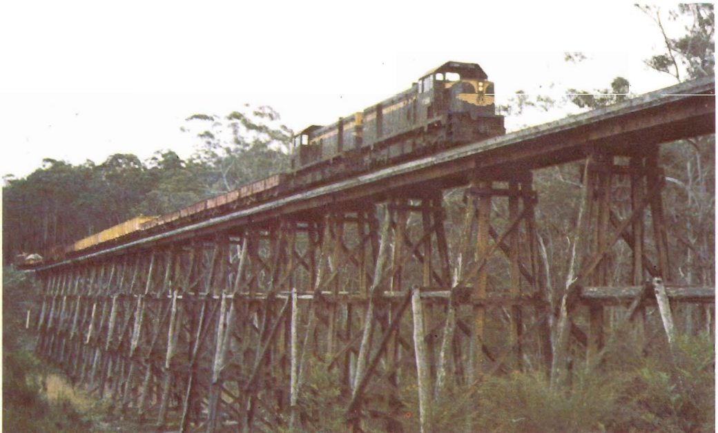
This handsome photograph, taken by Mr. T. V. Broderick of Dallas, Vic. shows two T class locomotives on an Orbost bound goods train crossing the Stony Creek trestle bridge at mileage 204. 66 on the upside of Nowa Nowa. The bridge, built in 1916, has 27 nine metre spans and is 247 metres long.
