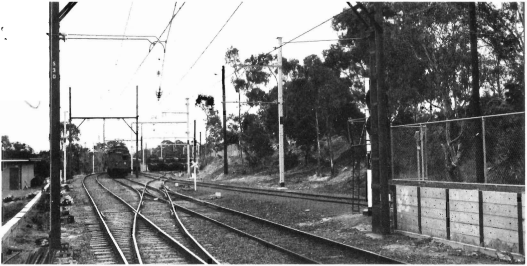
As a Hurstbridge bound train enters Macleod, it passes three Harris trains in the new stabling sidings.
