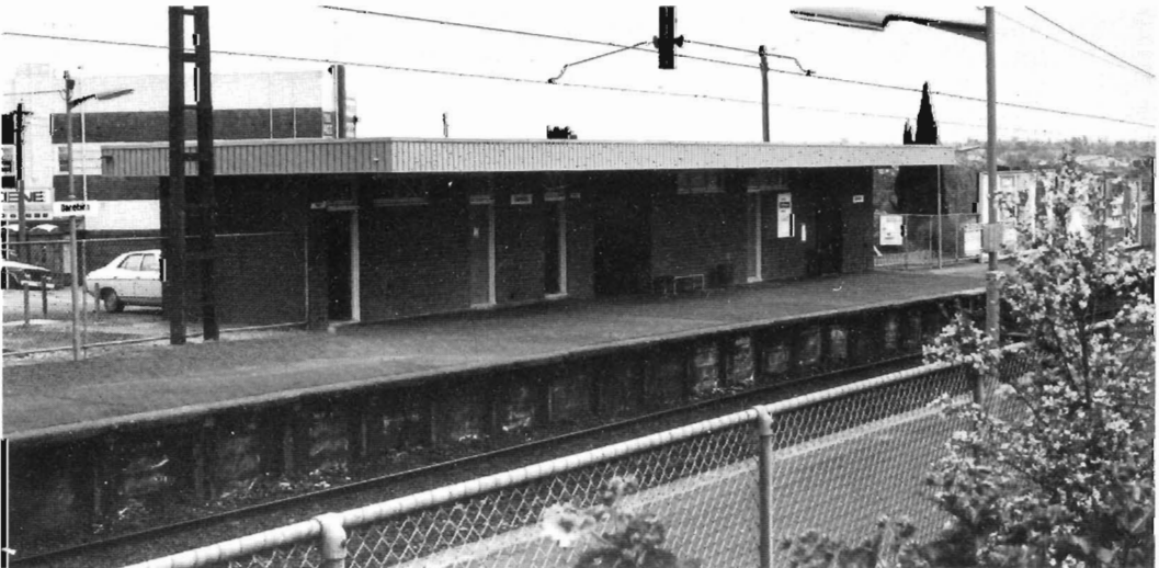
This new brick station building at Darebin has replaced an old wooden building.
