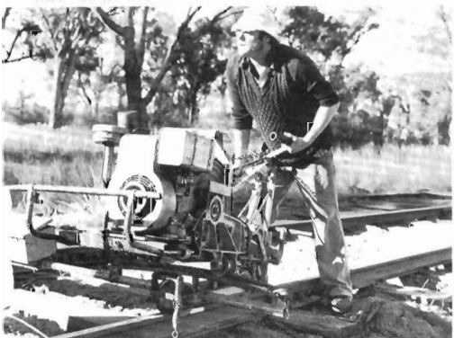
Hand tools such as the Nordburg wrench then removes the nuts and washers on the rail.
